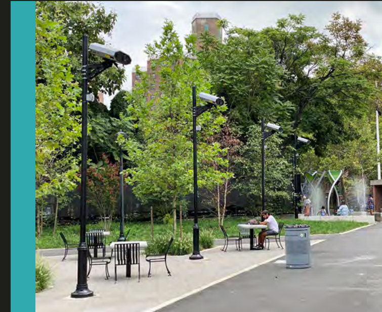
Pole mounted projectors
