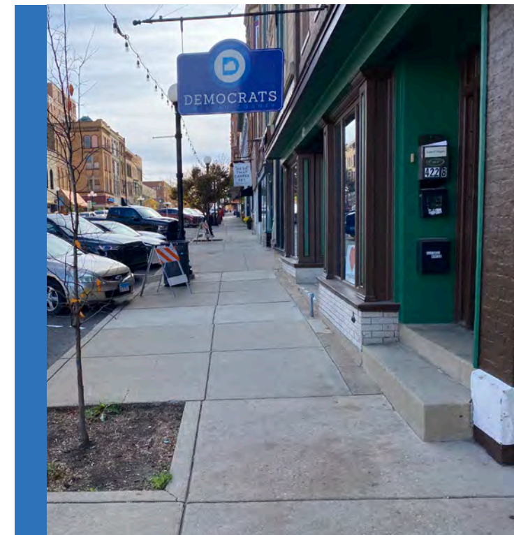
A row of inaccessible building entrances.
