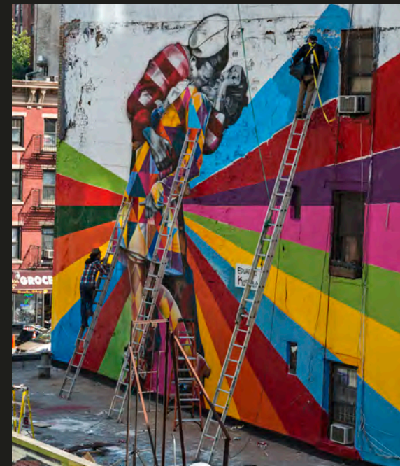
Murals can consist of paint applied directly to the wall combined with elements painted off-site to simplify the installation.
